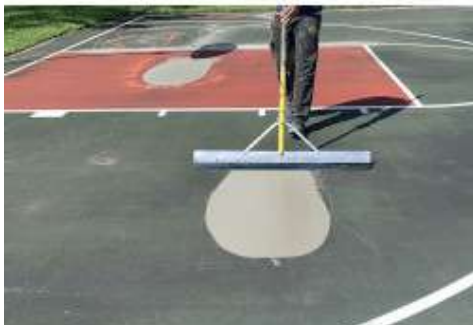
Use of ULTRABOND SPORT for levelling out depressions in the playing area
