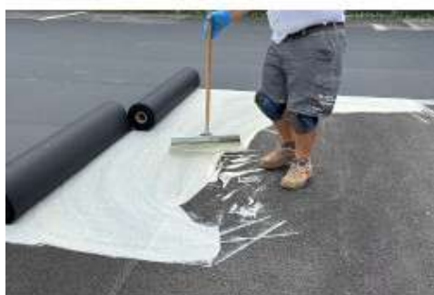
Use of ULTRABOND SPORT for bonding rubber mats, such as Mapecomfort R and Mapecomfort PU
