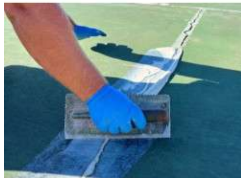
Using ULTRABOND SPORT for crack sealing
